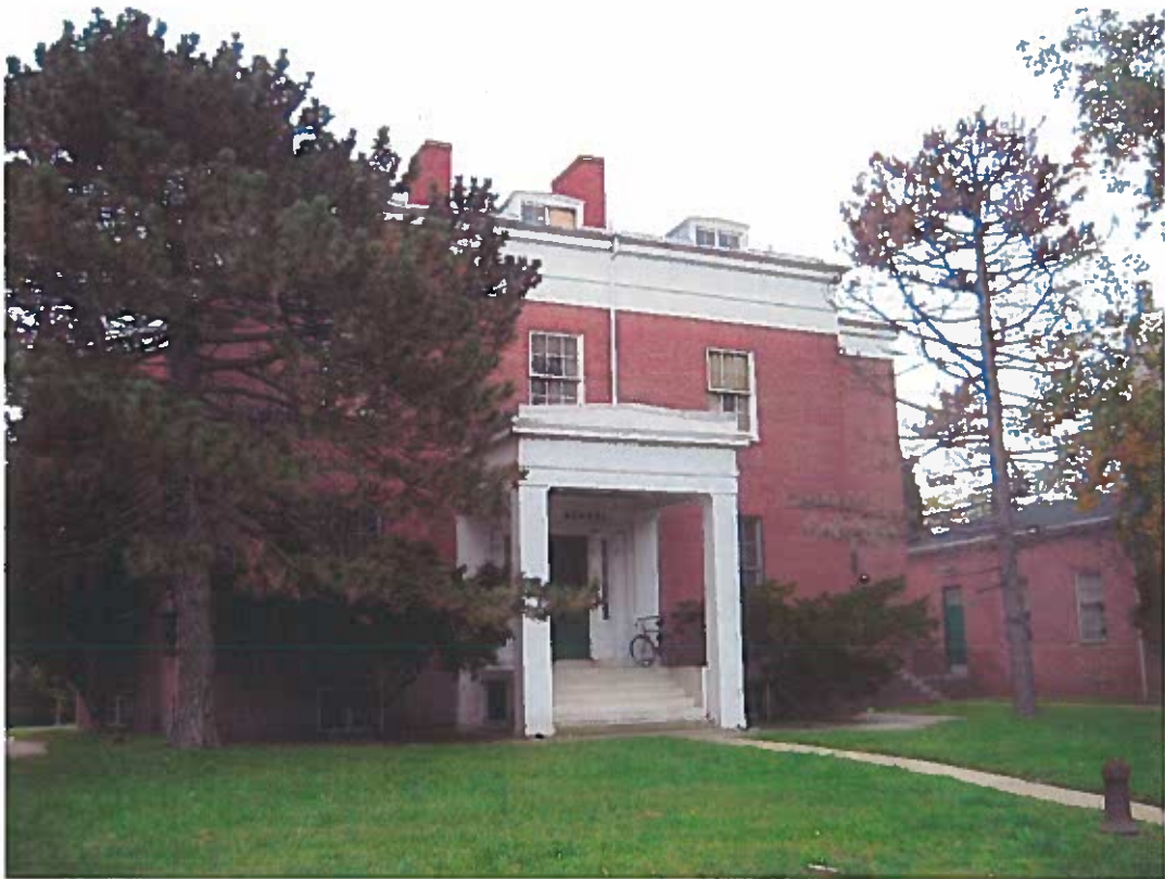
Front 1936 HABS Photo and Same View Today
