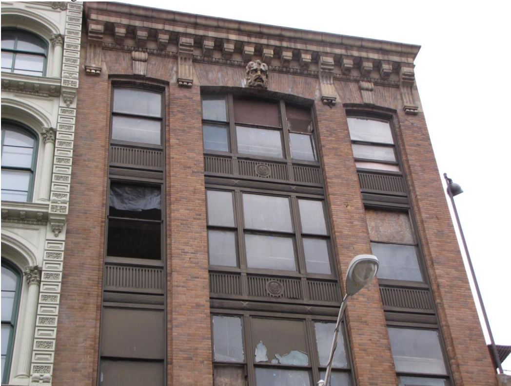
The upper floors of the W. Baltimore Street façade.
