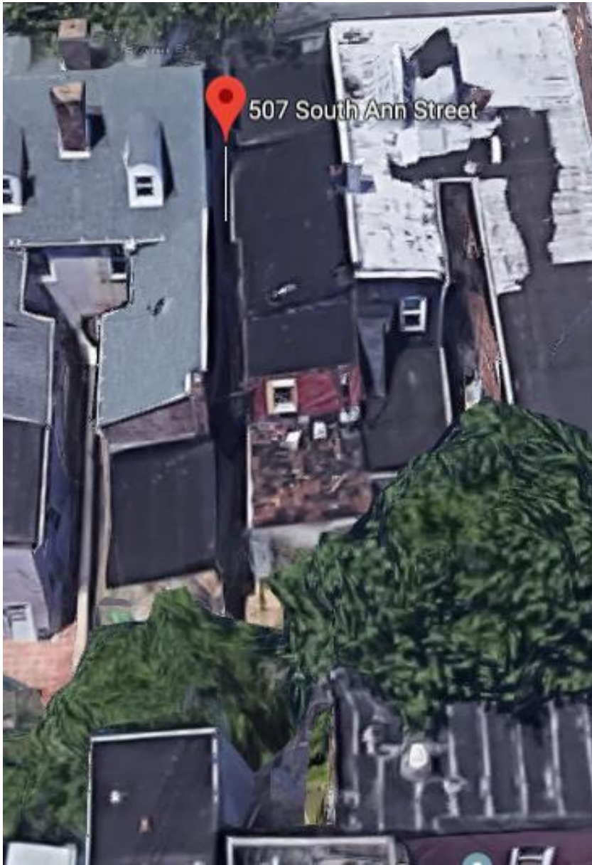
View from East of rear
