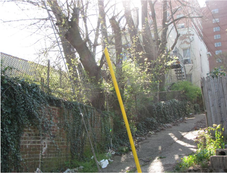
View of the rear of the Shelley house from “Shelley’s Alley”; facing west.
