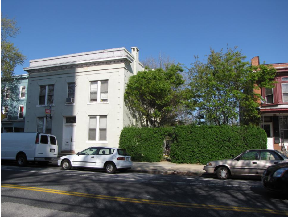
View of Shelley House and yard; facing east.
