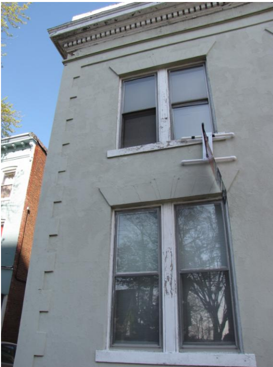
Detail of quoins and decorative jack arches.
