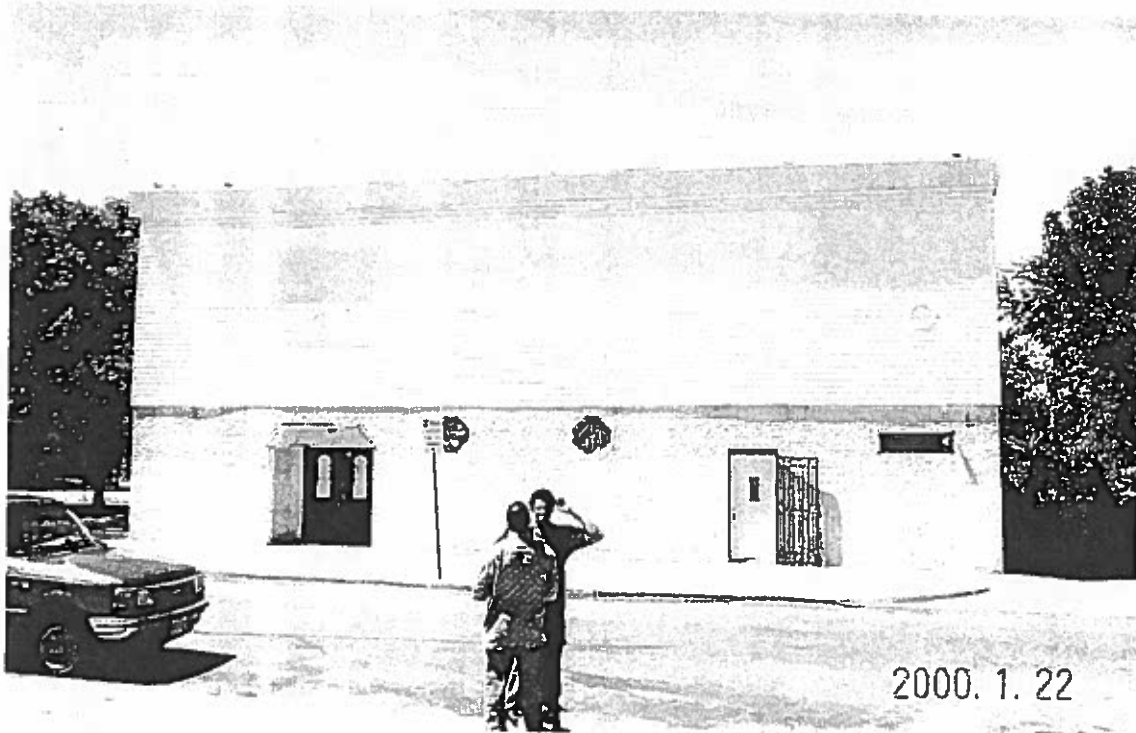
Front façade facing Islamic Way
