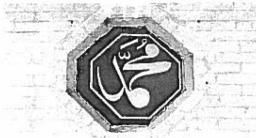
Window in Front Facade
