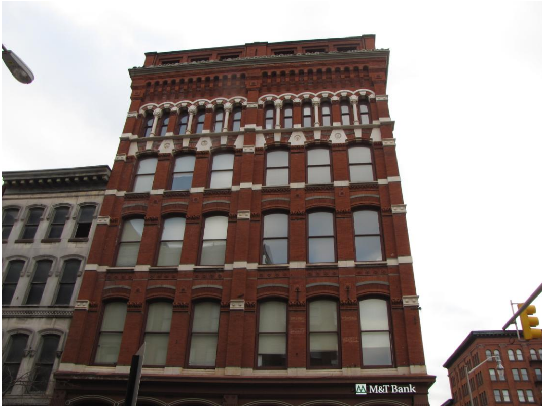
Upper Floors and Cornice, Baltimore St. façade.
