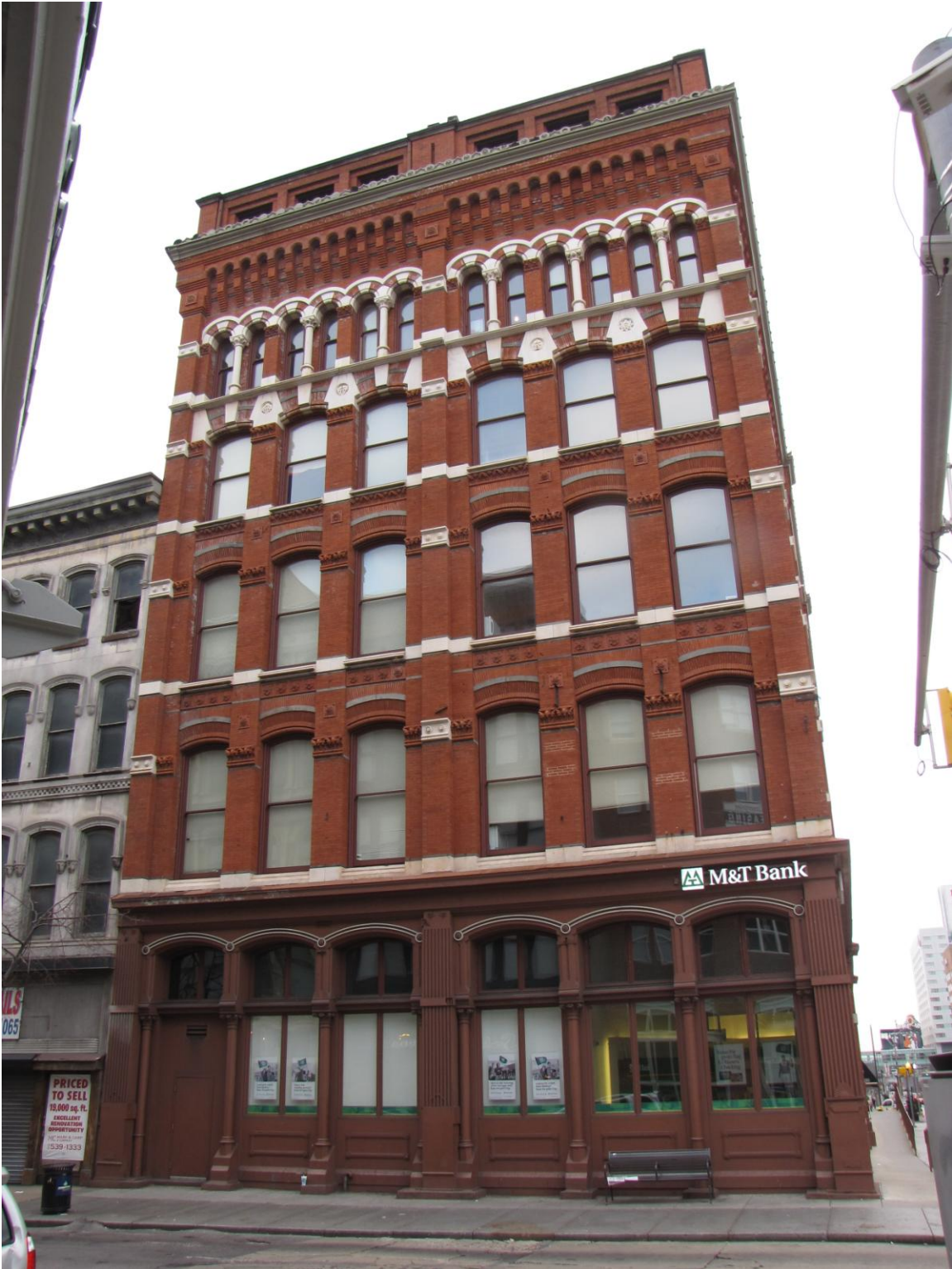
Baltimore Street façade.
