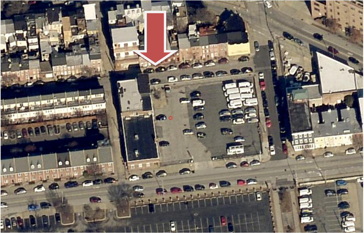
View from the South
