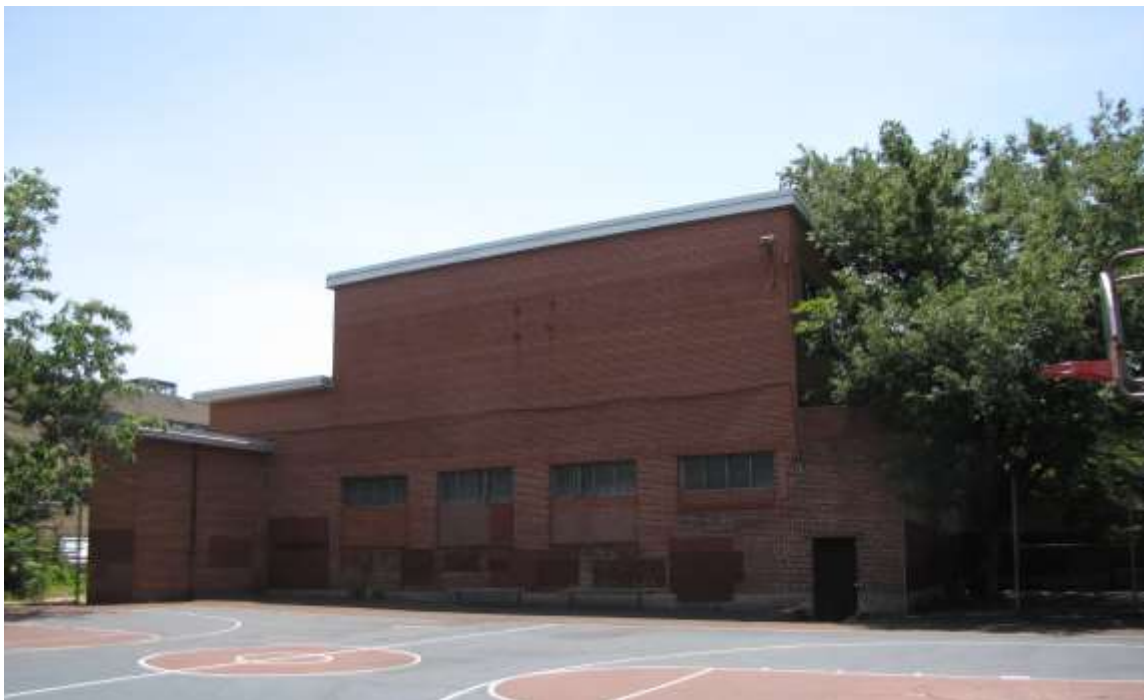
Image 4: North elevation of the swimming pool and multi-purpose room.
