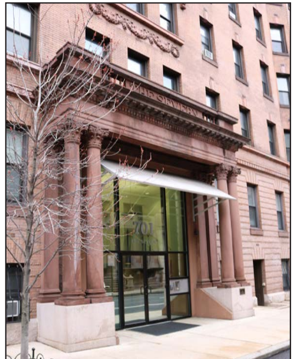
Figure 41: RECOMMENDED - Contemporary awning on non-original storefront. Not attached to historic material.
