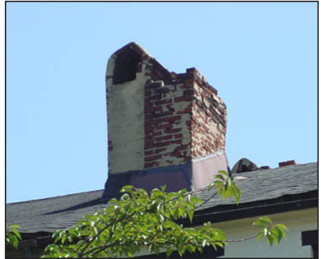
Figure 30: Example of chimney deterioration.
