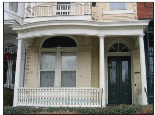
Figure 35: RECOMMENDED - Rehabilitated decorative wood porch.
