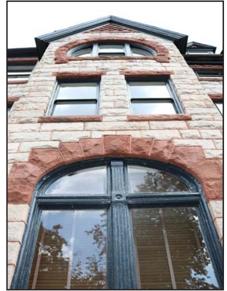
Figure 9: RECOMMENDED - Repointing of stone using appropriate mortar.
