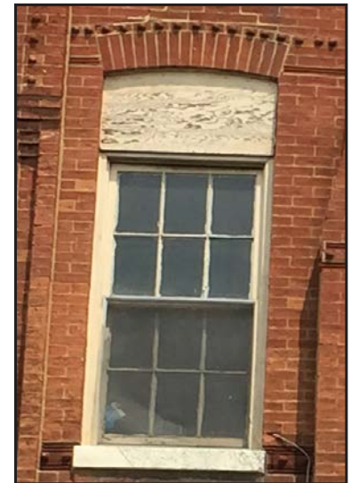
Figure 26: NOT RECOMMENDED An example of an inappropriate replacement window.
