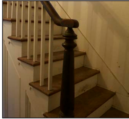
Right to left: Decorative wood floor, decorative wood newel post and balustrade, tile vestibule wall finish typical in many Baltimore rowhouses.
