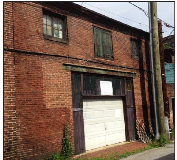
Figure 37: NOT RECOMMENDED - Inappropriate garage door infill.
