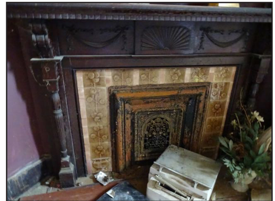
Figure 60: NOT RECOMMENDED - Historic fireplace with various deteriorating materials.
