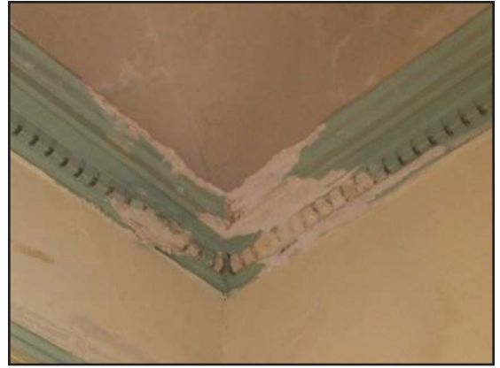
Figure 61: Deteriorating decorative plaster trim.
