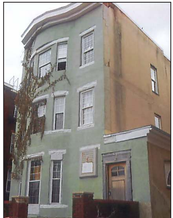
Figure 6: NOT RECOMMENDED - Inappropriate use of stucco on an historic masonry building.
