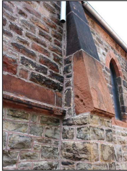
Figure 8: NOT RECOMMENDED - Discoloration and deterioration of historic stonework due to water damage.
