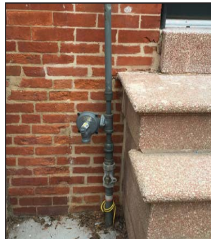
Figure 1: NOT RECOMMENDED - Example of brick wall with deteriorating mortar, water damage, and inappropriate repointing.
