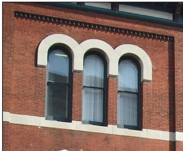
Figure 23: RECOMMENDED - Example of appropriate replacement windows.
