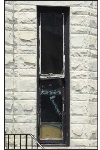
Figure 25: NOT RECOMMENDED An example of a window that is deteriorated beyond repair.
