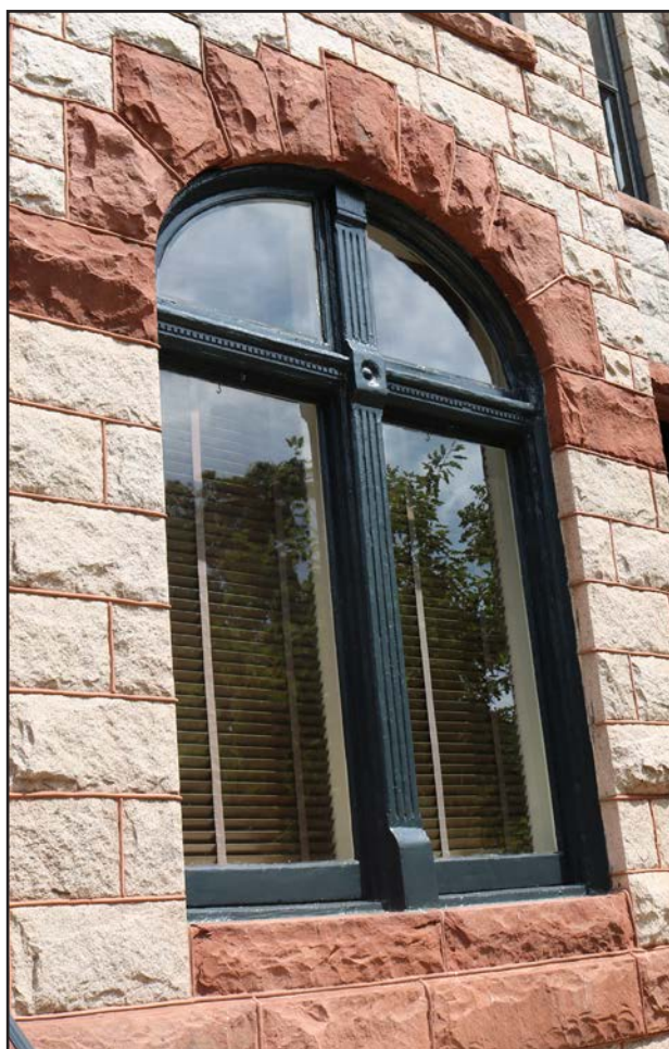
Figure 24: RECOMMENDED - Example of appropriate repair of historic wood window.
