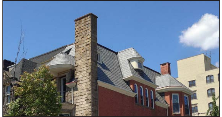
Figure 29: RECOMMENDED - The deteriorated slate roof was replaced using Tru-Slate, an innovative option when slate replacement is required.
