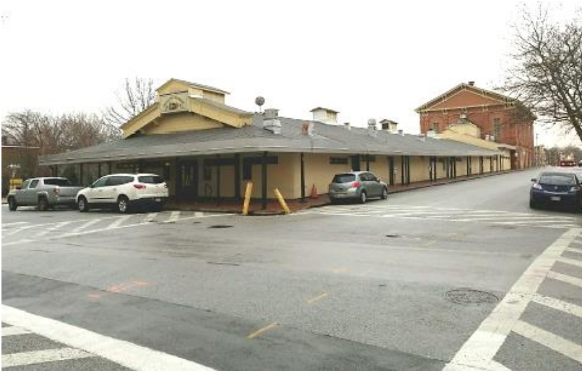
Image 9: 26 S. Arlington Avenue, Hollins Market shed looking west – Existing conditions
