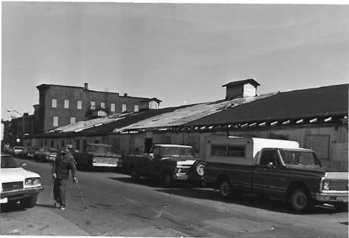
Image 8: Hollins Market shed looking east, April 10, 1979
