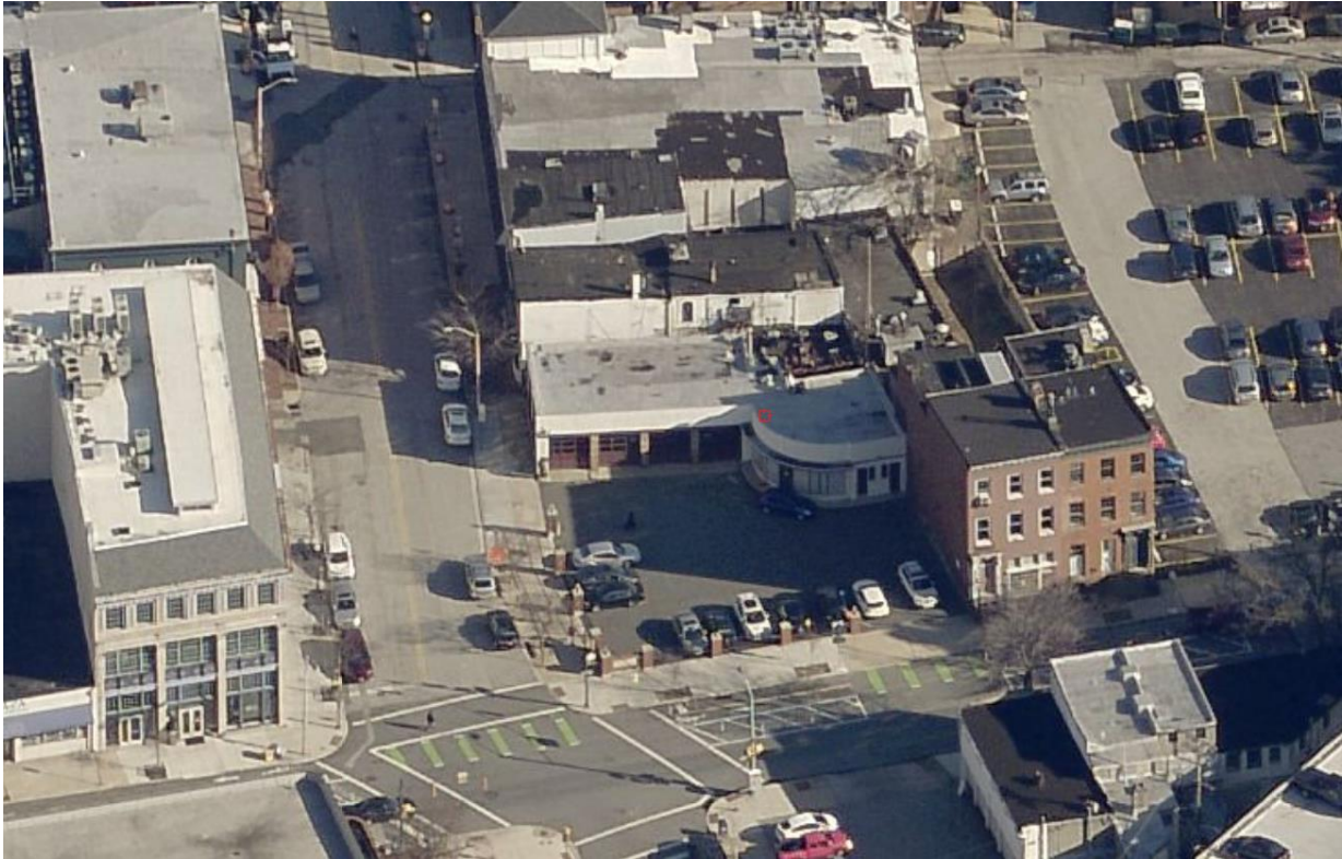
Image 3 –Aerial view of building from west.
