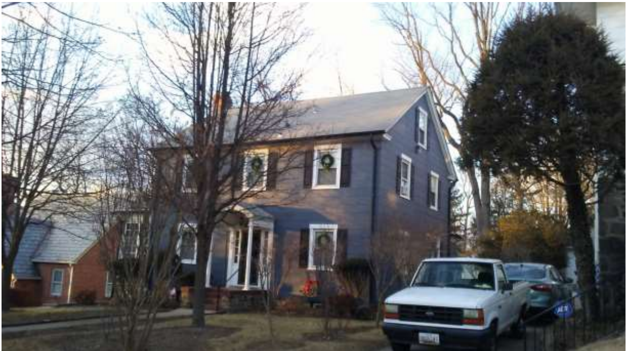
Image 5 –View of front and east elevation, from sidewalk.
