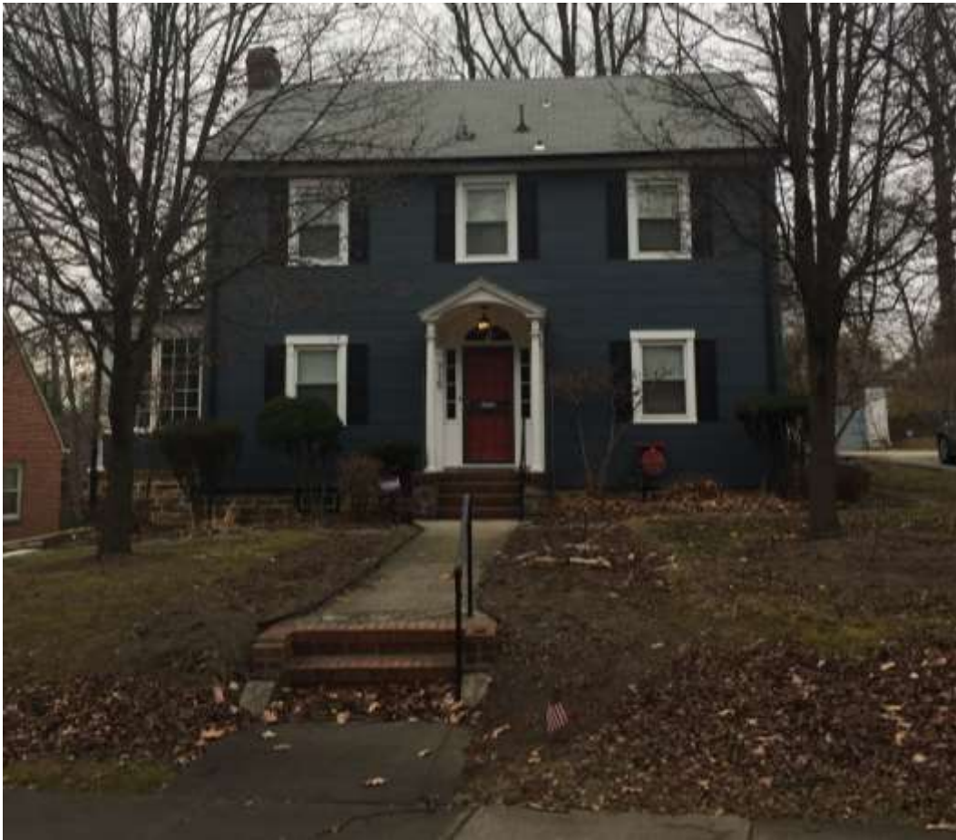
Image 3 –View of front elevation.
