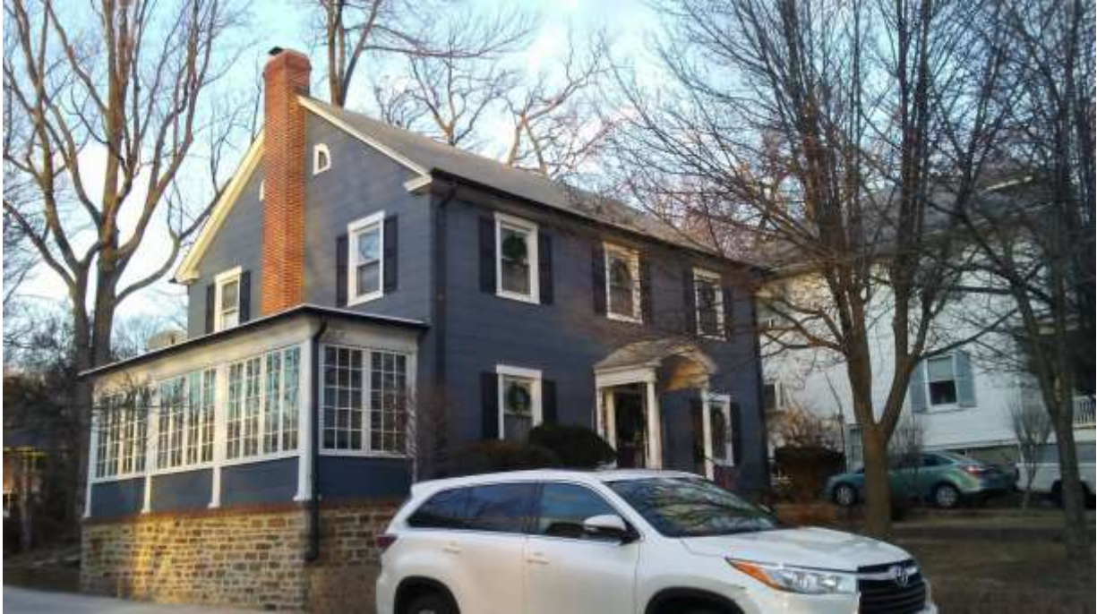
Image 4 –View of front and west elevation, from sidewalk.
