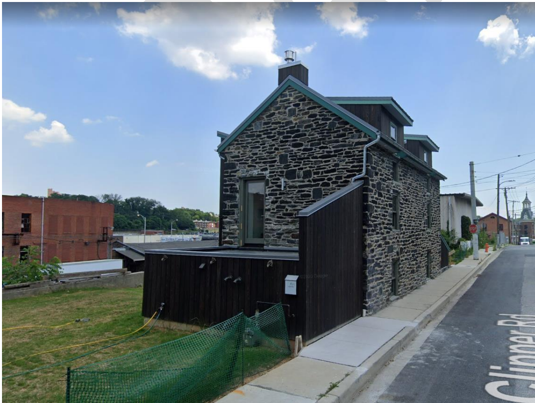
Image 2: 3605 Clipper Road site – Google streetview image of renovated main building at the site.
