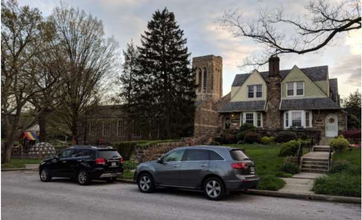
Image 6: View of Norman Ave. façade, from sidewalk on Norman Ave.
