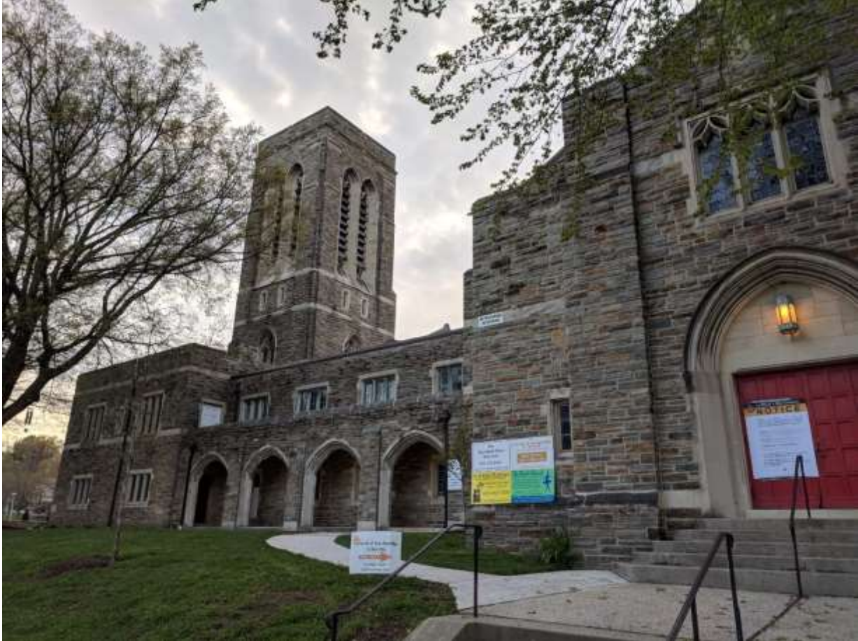
Image 4: View of Norman Ave. façade, from sidewalk on Norman Ave.
