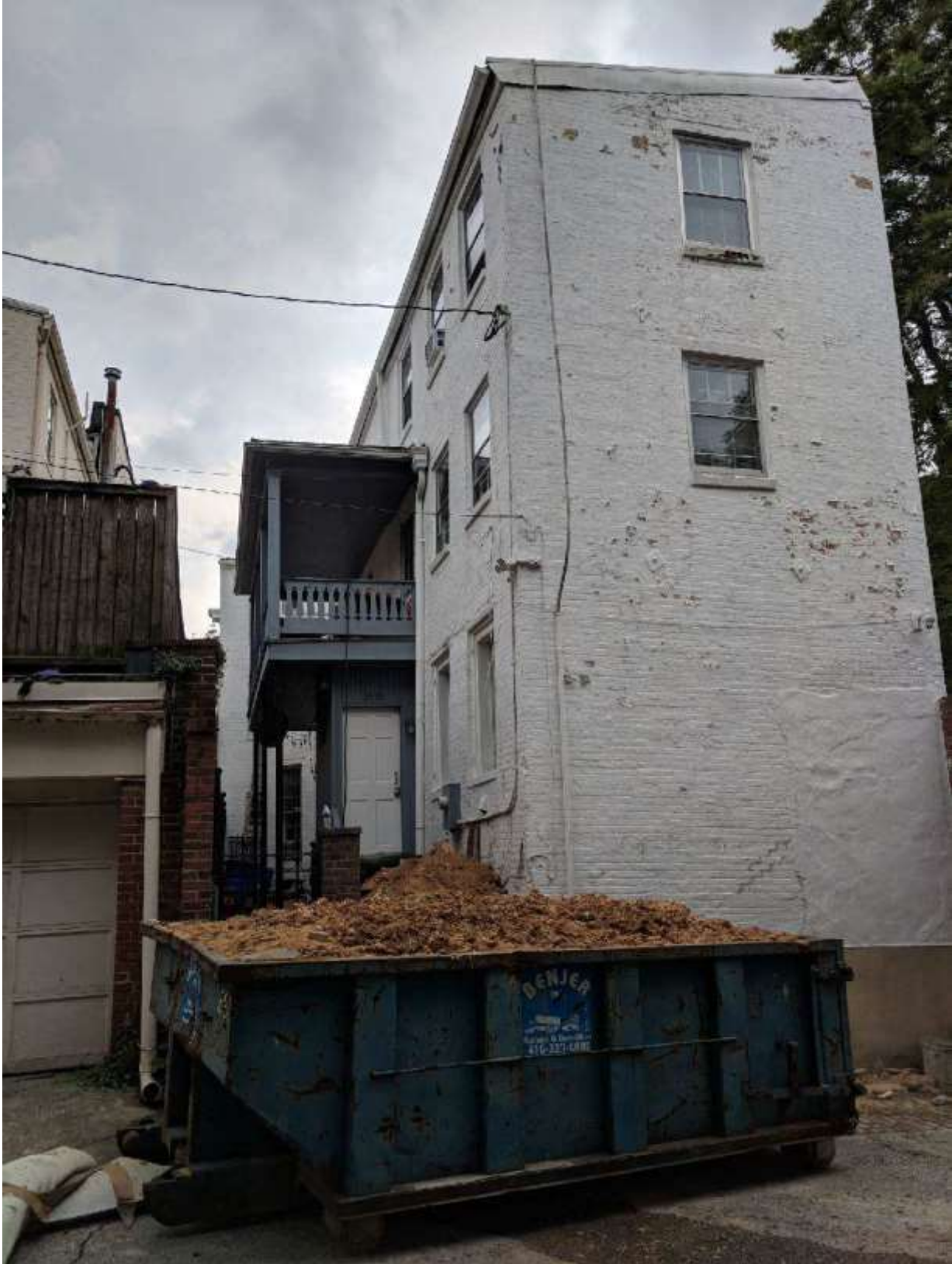
Image 7: Rear elevation from Jordan Street.
