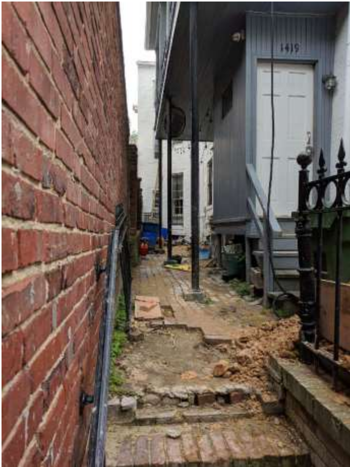
Image 10: The remaining 15 windows located on the rear and side elevation are not highly visible from Jordan Street. This view is from the back gate of the property. The windows at the rear are the same as in Image 6.
