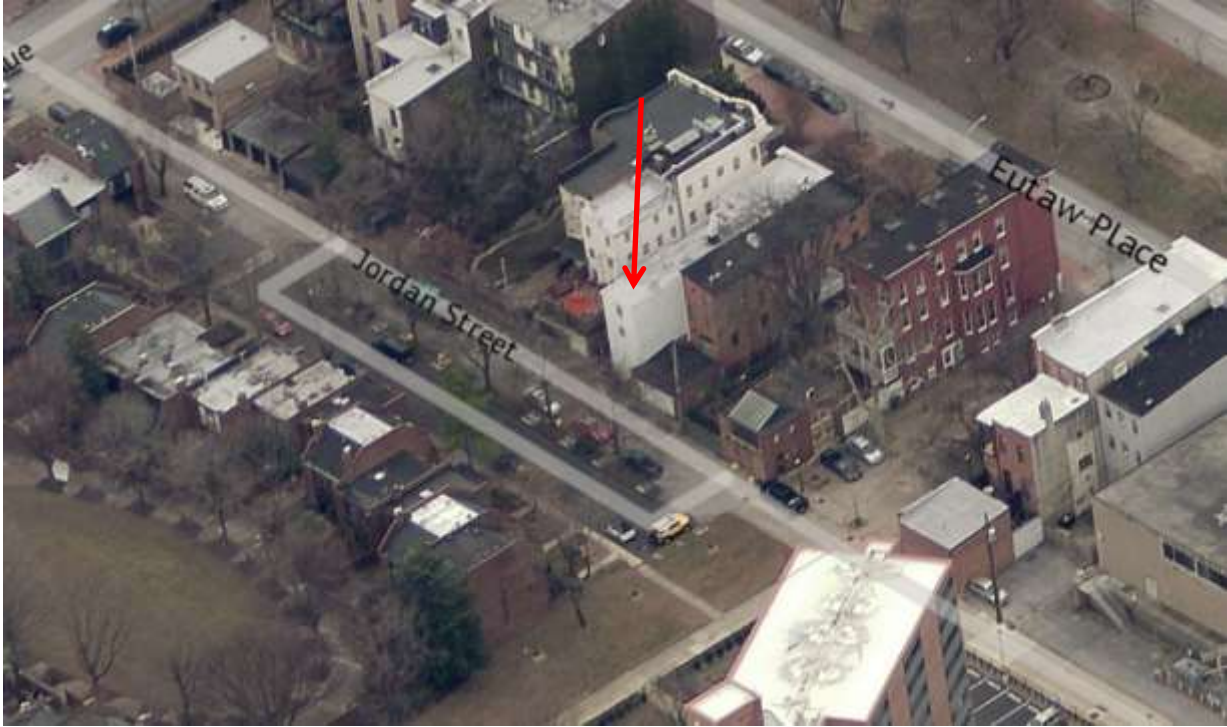
Image 3: Aerial view of the property from the north.
