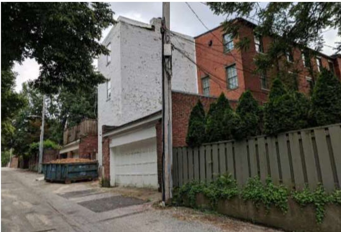
Image 11: Contextual view of Jordan Street, showing the rear of the property and neighboring 1421 Eutaw Place.
