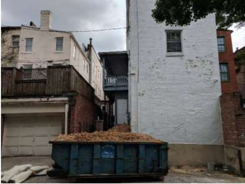
Image 9: Rear elevation from Jordan Street, highlighting the 10 windows that are highly visible from this public right of way.
