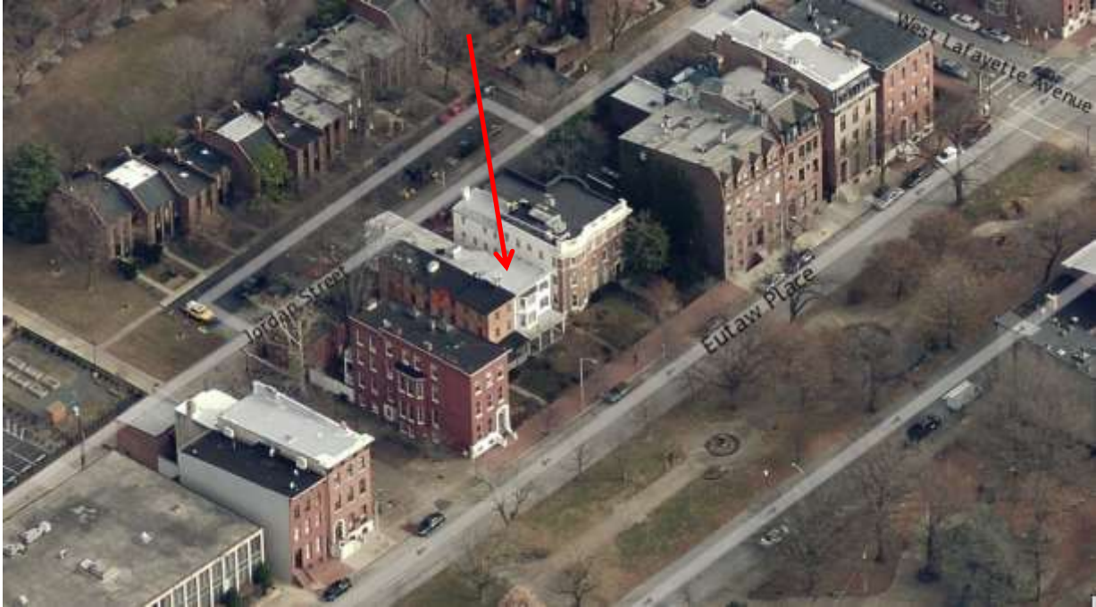
Image 1: Aerial view of the property from the west.
