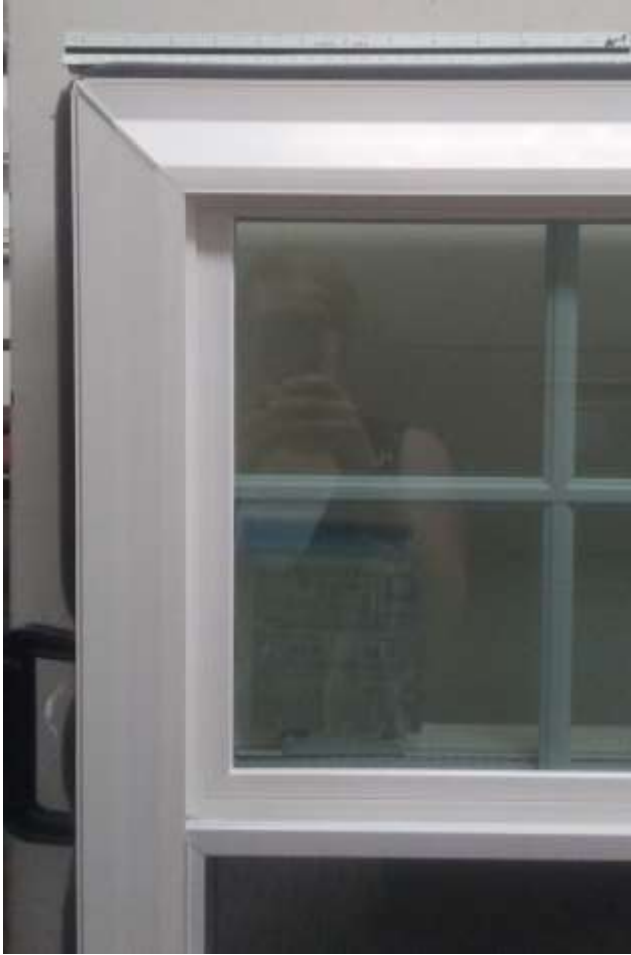
Image 14: Detail of window frame.
