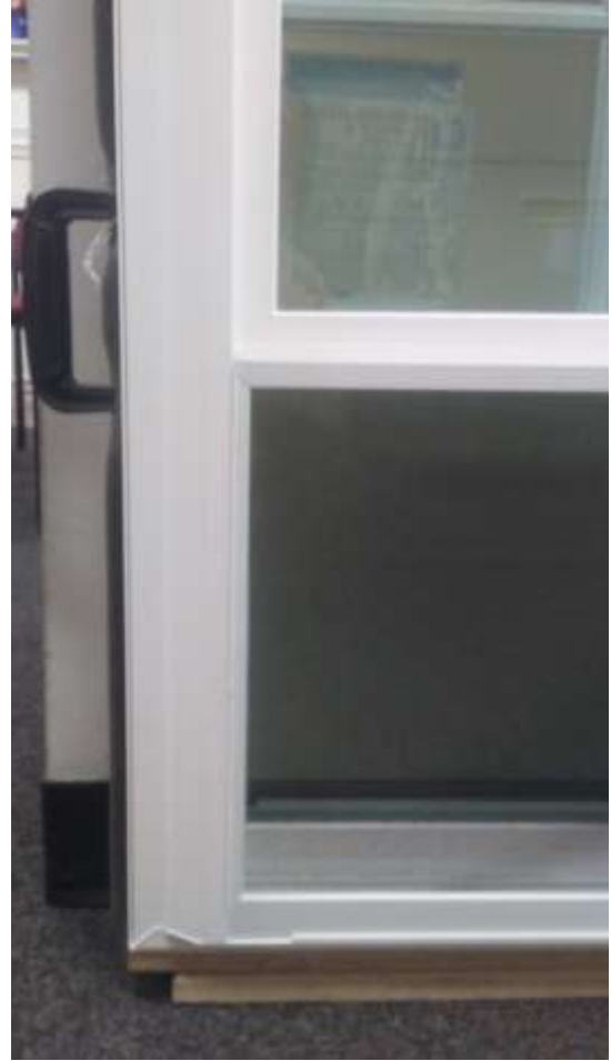
Image 15: Detail of window base.
