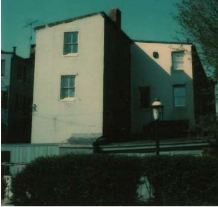
Image 5: Polaroid of rear elevation, undated. Note the 2/2 windows on the rear elevation, as well as the wooden wall and small rear addition. (All of which were removed without CHAP review at some point in the last 50 years)
