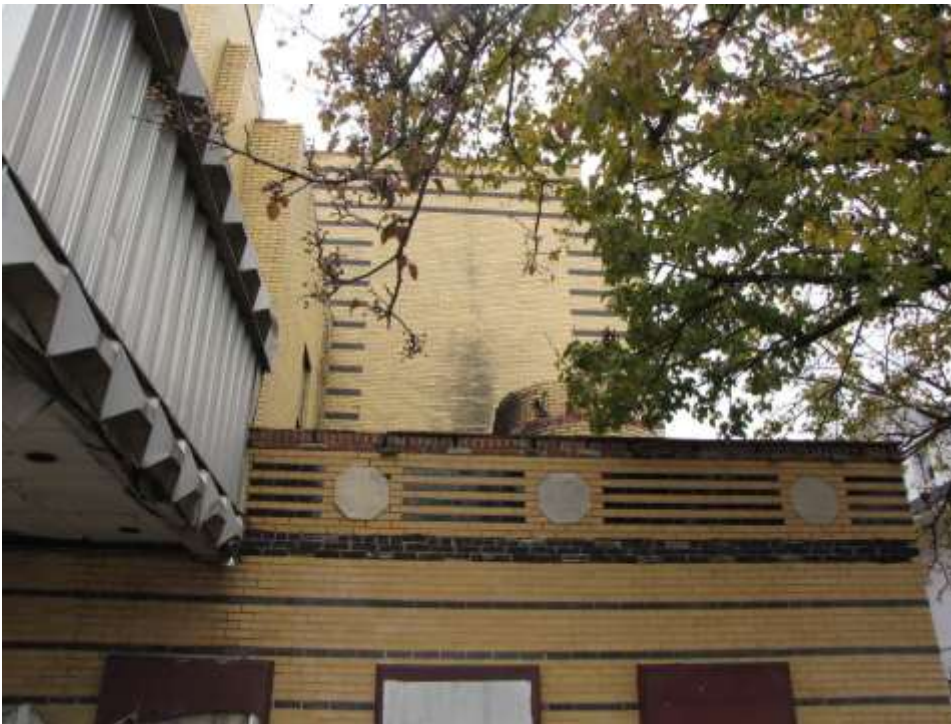
Detail of Cornice in November 2013.
