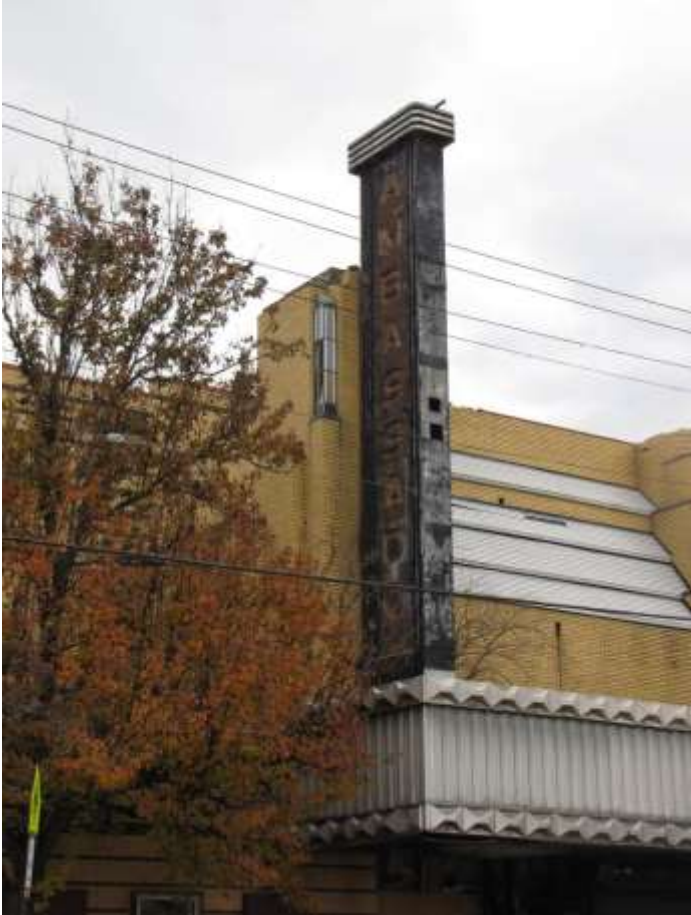
Detail of marquee in November 2013.
