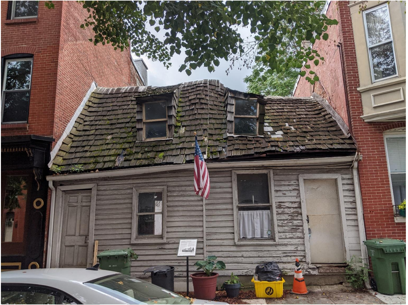
Image 4: 612-614 South Wolfe Street façades, July 2020
