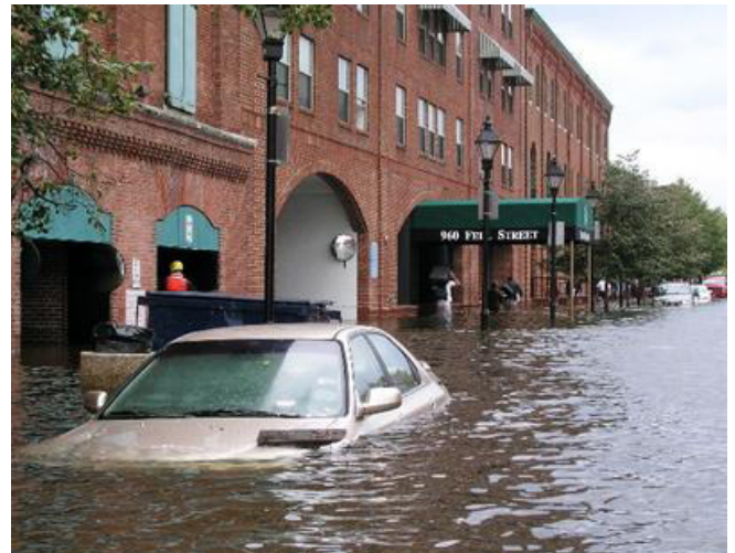
Henderson's Wharf experienced severe flooding as a result of Hurricane Isabel in 2003. (Source: Baltimore Office of Sustainability.)
