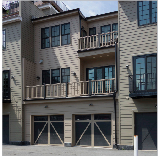
The front elevation (at left) of this wet floodproofed rowhouse maintains its historic character. At the time of renovation, it was missing its rear wall, providing a unique opportunity for substantial alterations. The contemporary rear elevation (at right), includes a roof deck, balcony, and garage door openings. The basement has been infilled and first floor uses limited to an entrance, garage, and storage space.
