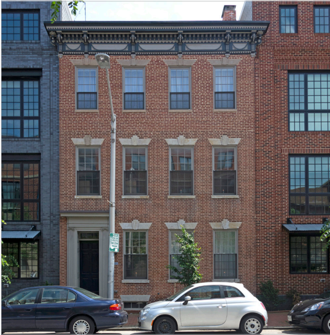
The front elevation (at left) of this wet floodproofed rowhouse maintains its historic character. At the time of renovation, it was missing its rear wall, providing a unique opportunity for substantial alterations. The contemporary rear elevation (at right), includes a roof deck, balcony, and garage door openings. The basement has been infilled and first floor uses limited to an entrance, garage, and storage space.
