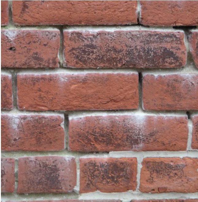
Repointing of open joints can reduce interior damage from wind-driven rain and floodwater.
