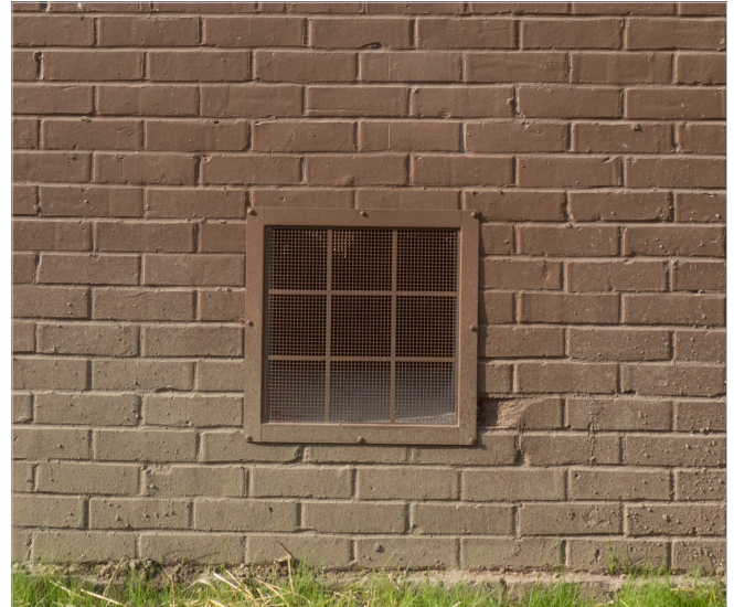
Flood vents are a key element of wet floodproofing. By painting it to match the adjacent wall color, this flood opening is less visually obtrusive.
