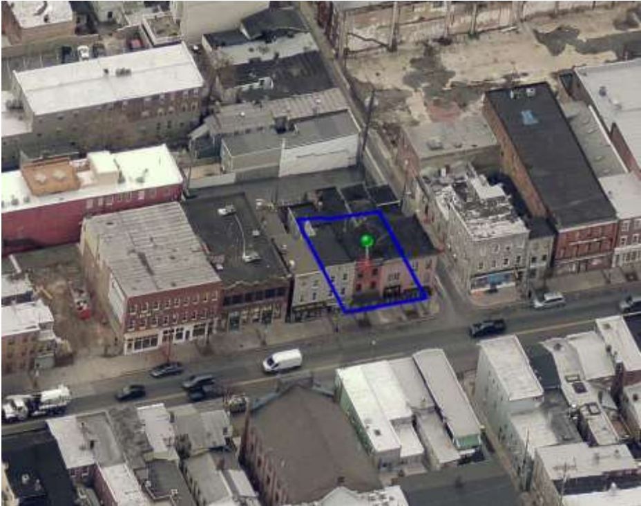
View from North
